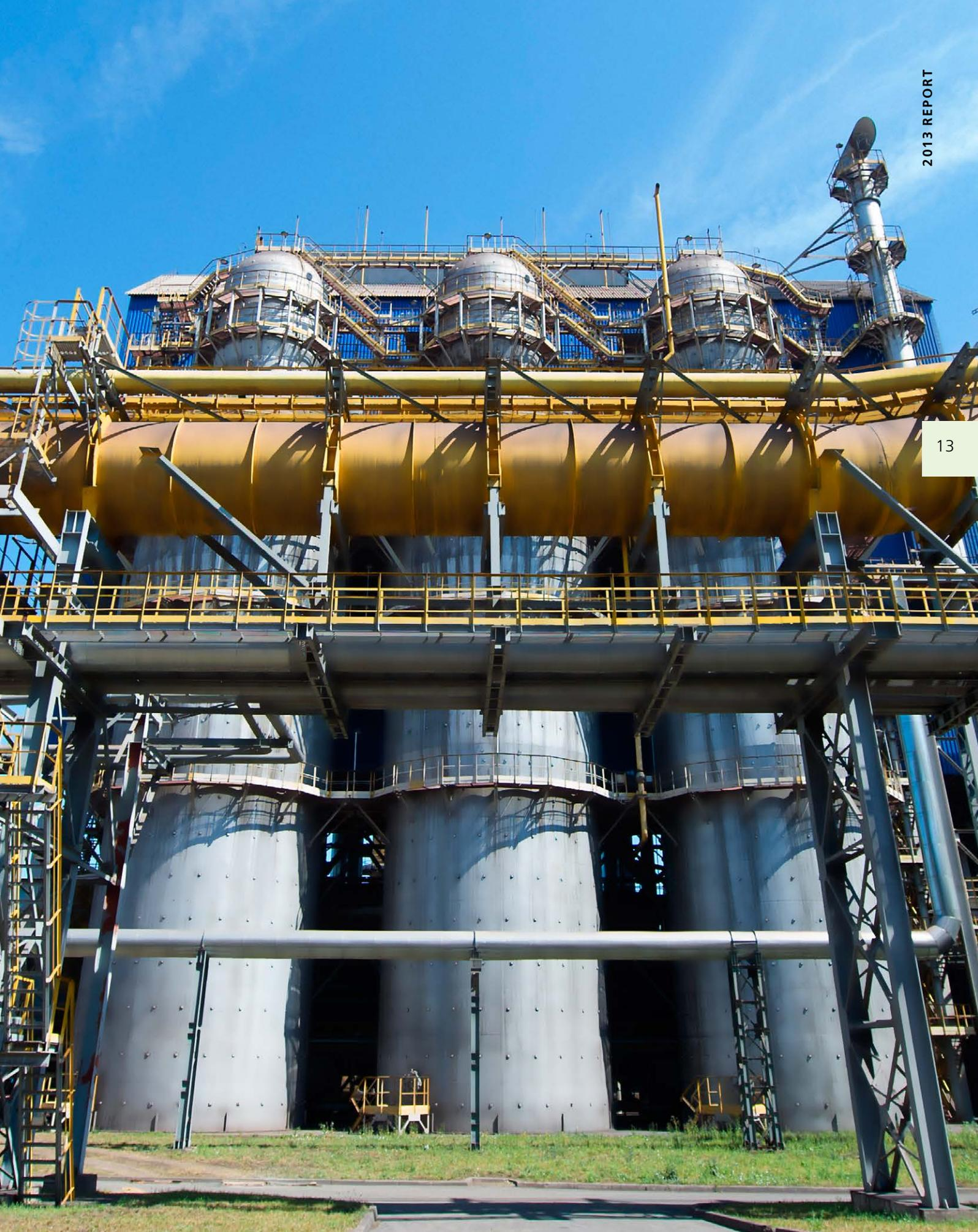
↑ In the photo: the use of shaftless hot blast stoves at Blast Furnace #7 has allowed for the reduction of carbon oxide emissions by several hundred times.
