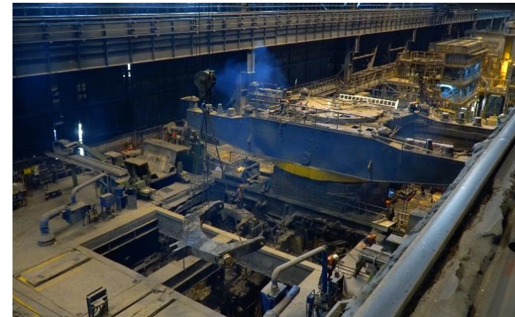
NLMK Lipetsk: CCM#9 assembling works
